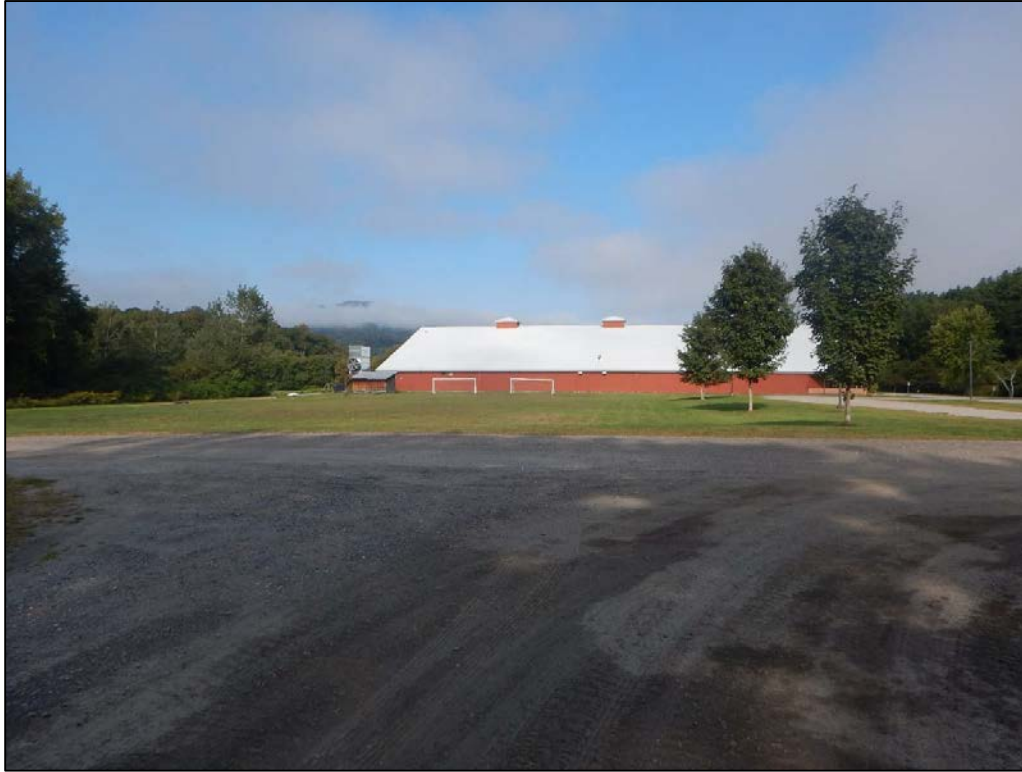
Photo 8. Ice Center property, note ice center building in the background and gravel parking area. View to the northwest.
