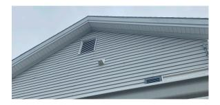
Soffit will match existing soffit, See picture of current white 4" soffit: (Also Shown in Above Picture.)
