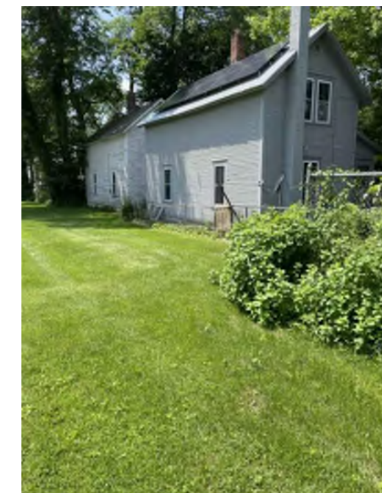
EXISTING NW PERIMETER
