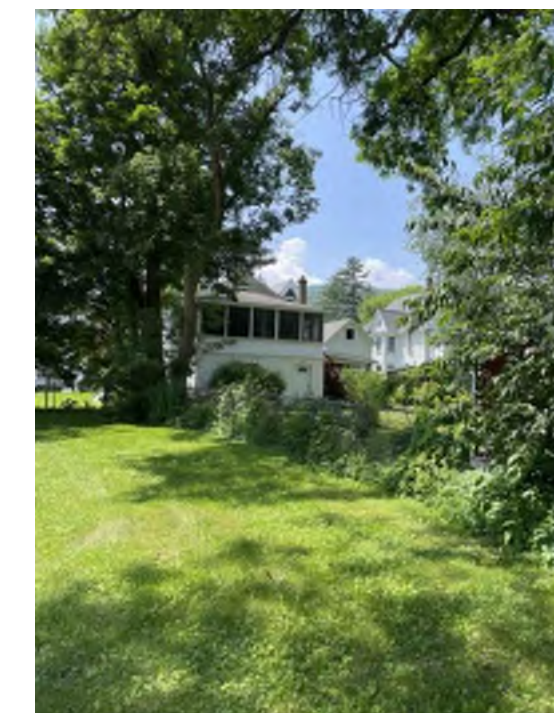
EXISTING NW PERIMETER
