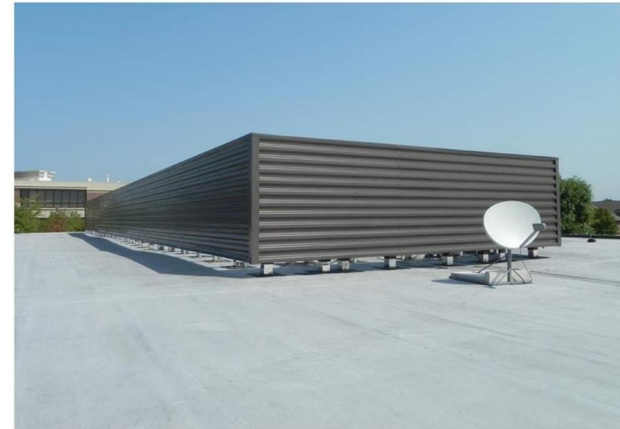
The 7.2 Rib panel in a horizontal application with 5x5 corner trim.
