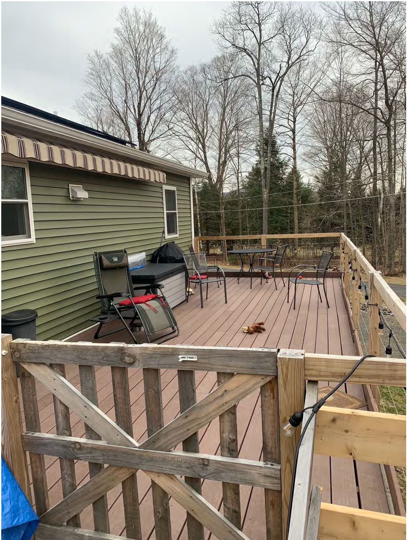
Looking South from the landing at the top of the stairs.
