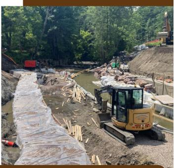
The cast-in-place concrete footing being kept wet during the cure period and an excavator building the crane pad for the 450-ton crane.
