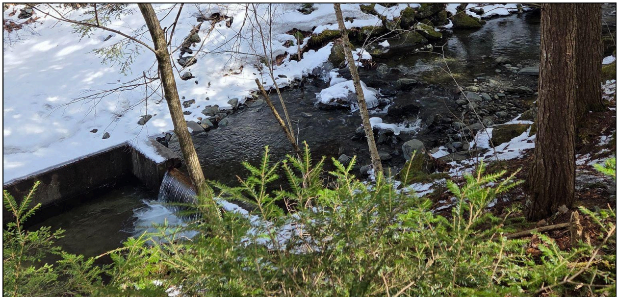
Figure 28, below: EFUD infrastructure along Tyler Brook.
