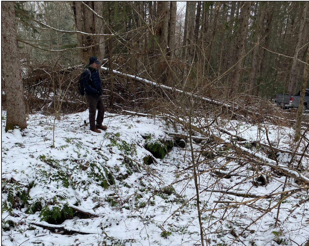
Figure 10: Foundation 1, referenced in Figure 9 above.
