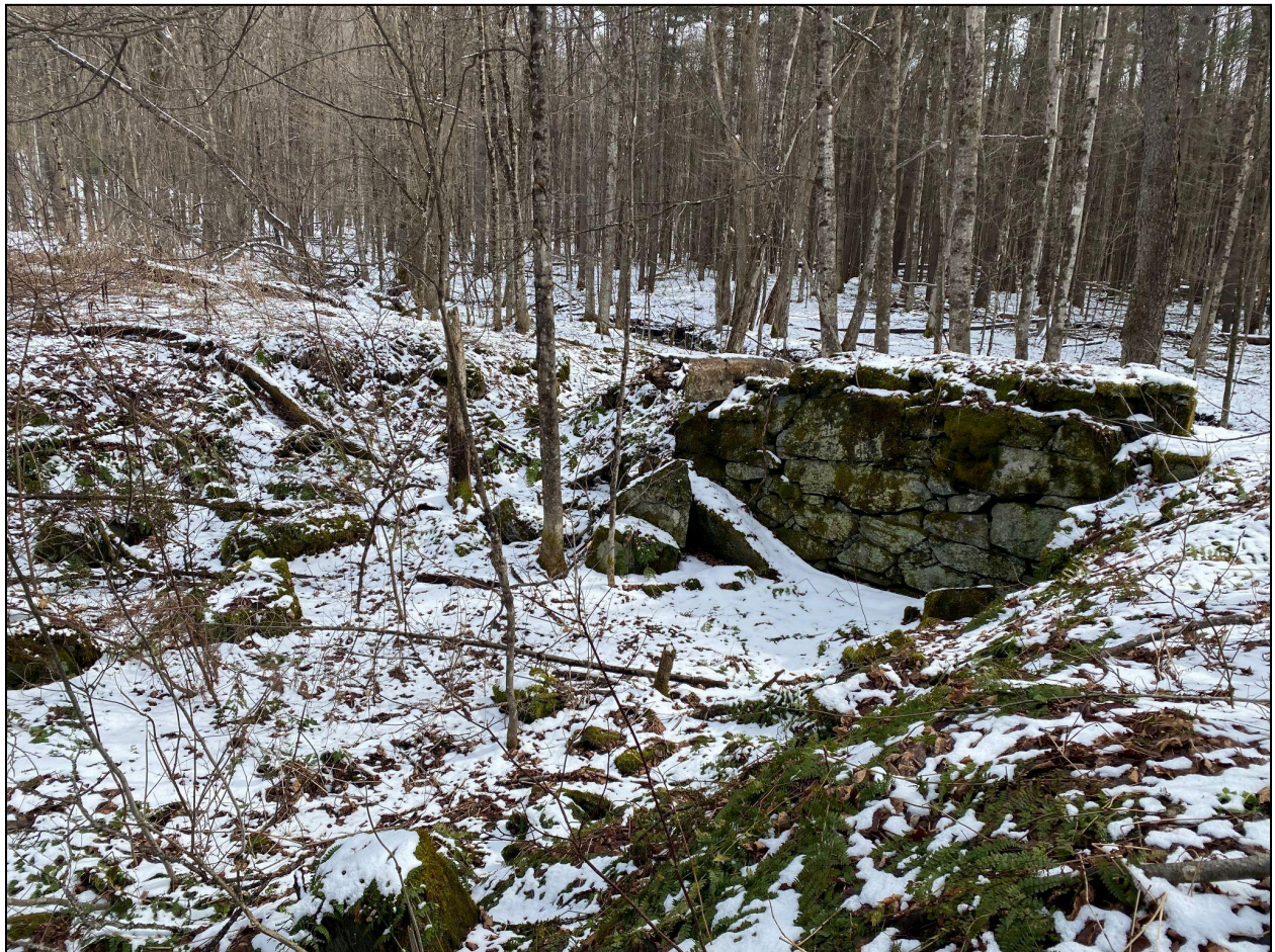
Figure 12: Foundation 3, referenced in Figure 9 above.
