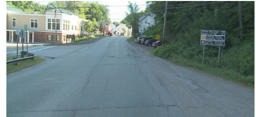
Stowe Public Safety Building at northern end of project area.
