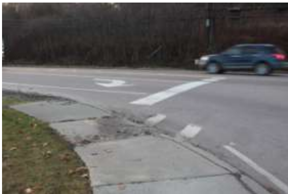
Poor drainage at the Shaw's driveway intersection
