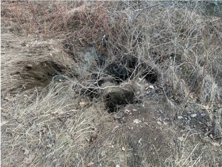
Surface of the leak
