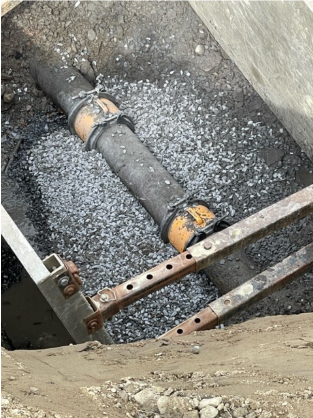
After the repair
