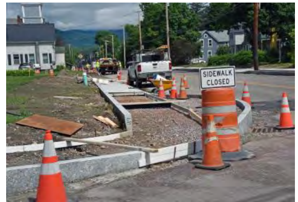
Main Street Reconstruction circa June 2020. Photo: Gordon Miller (provided by Revitalizing Waterbury).
