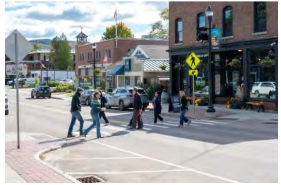
Pedestrians using a Main Street crossing with traffic calming bumpouts created during the Main Street Reconstruction project. Photo: Bobbi LoCicero (shared by Vermont Natural Resources Council).
